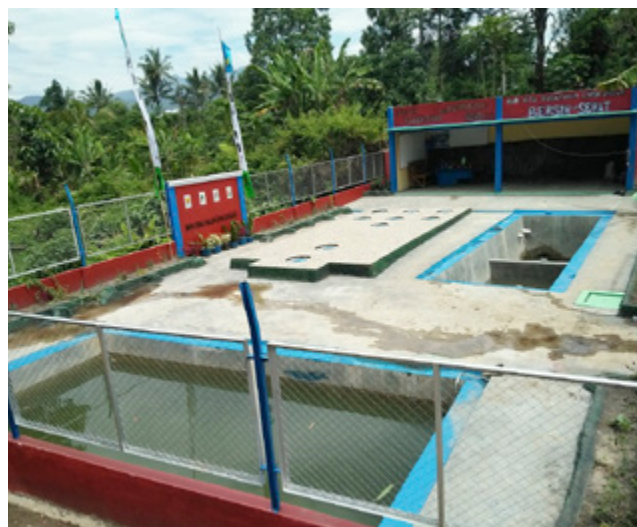
Waste treatment plant with balancing pond
