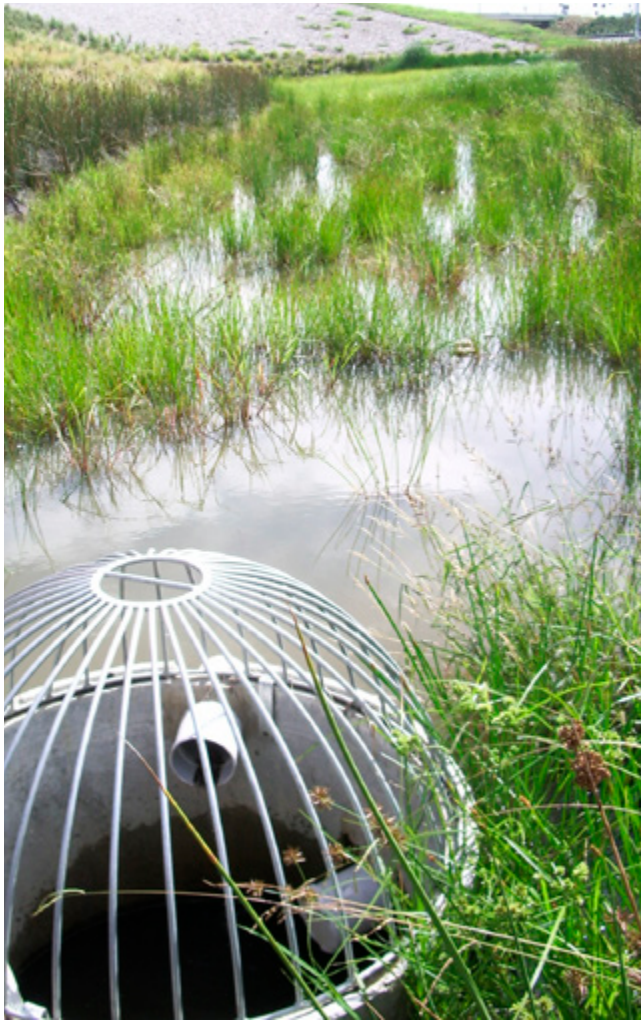
Raingarden (top) and constructed wetland (above) — two examples of green infrastructure used to manage stormwater in Water Sensitive Urban Design
