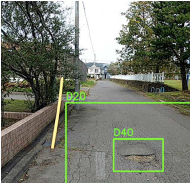
Road damage detected by smart phone using deep learning. Clockwise from top left: D00: linear crack; D20: alligator crack; D43: white line blur; D40: pothole
