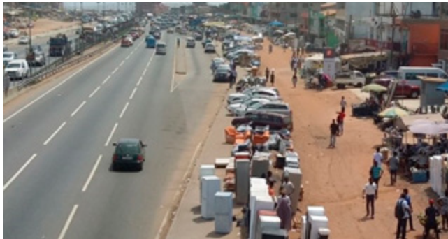
Section of the N1 Highway in Accra with pedestrian pavements encroached on by traders
