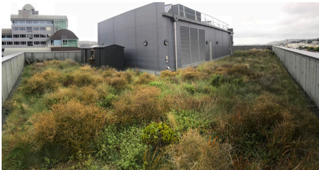
Green roofs are one instance of green infrastructure used to manage stormwater in Water Sensitive Urban Design
