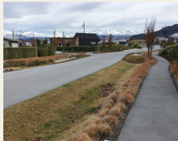
Kirimoko Park, with grass swale for managing stormwater
