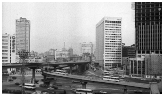
Old Seoul station overpass
