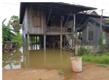
Annual flooding events leading to overflowing septic tanks
