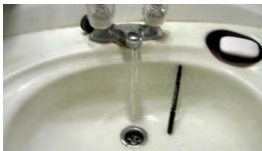
Device of saving water to adjust width of water flow from a tap as same as pencil
