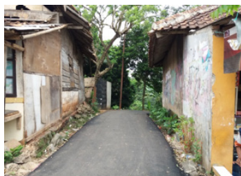
The poor settlement (2-5%)
